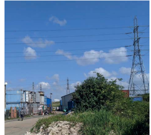
Figure 33: Large Scale Pylons
