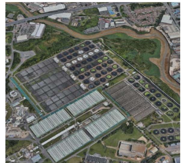
Figure 35: Beckton Sewage Works
