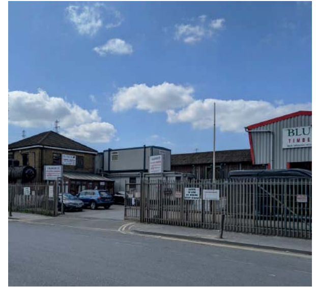
Figure 19: River Road looking South
