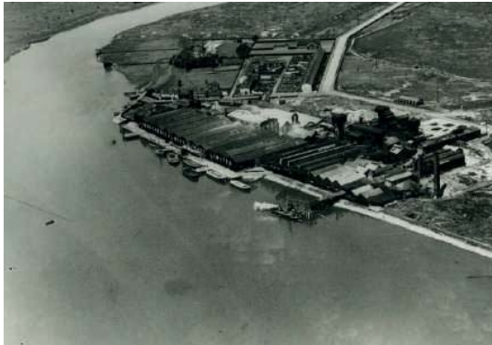
Figure 6: Aerial view of Lawes Chemical and Fertiliser Company
