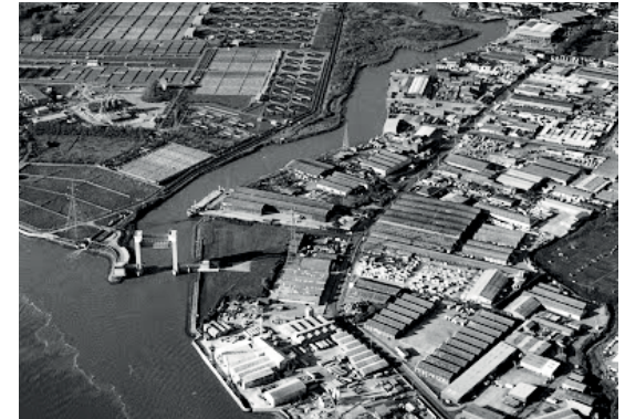
Figure 8: Aerial view showing Creekmouth Flood Barrier
